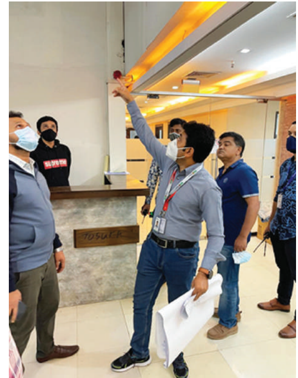
Photo: RSC's safety engineers verifying the installation of the fire pump (part of the Fire Suppression System) at an RSC-covered factory
