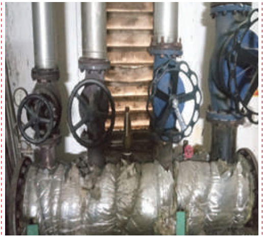
Safety valve's outlets are not directed to outside of the boiler room.
