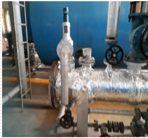
Safety valve's outlets are not directed to outside of the boiler room.
