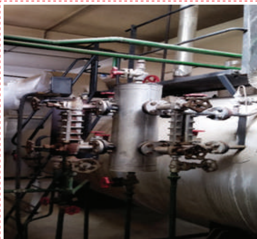
Indication of 'low low' water level is not identified.
